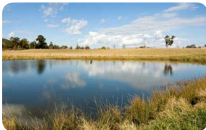
After using Aquatic Dam Stop Leak Professional
