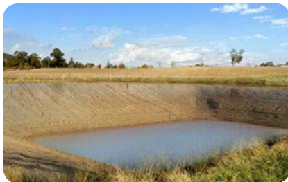
Before using Aquatic Dam Stop Leak Professional
